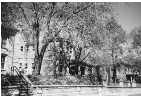
Historic mansions on Hall Street, St. Joseph, MO
