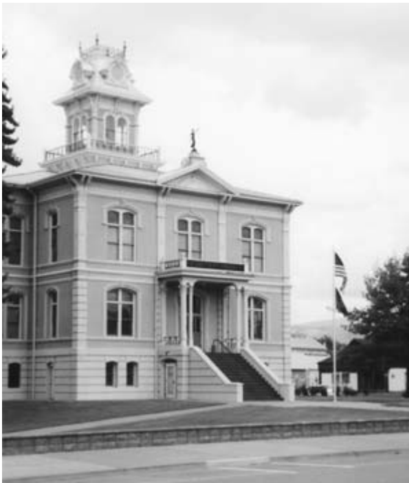
Columbia County Courthouse, Dayton, WA
