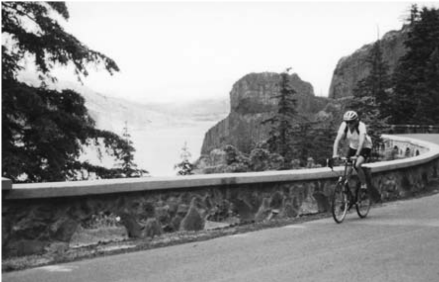
Historic Columbia River Highway
